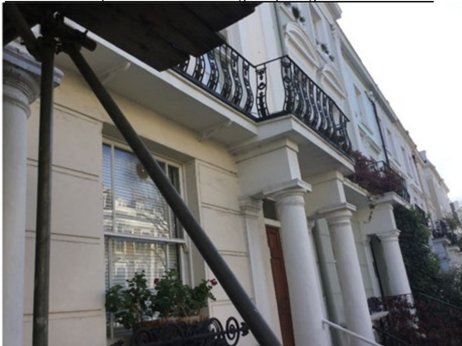
View of Balcony Structures of Buildings Adjoining to South of no. 23
