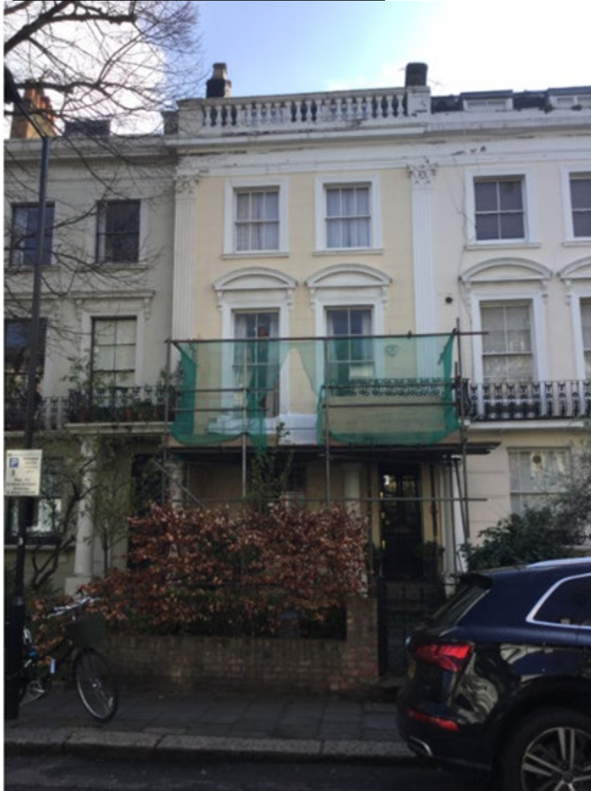
Front Elevation After Removal of Balcony
